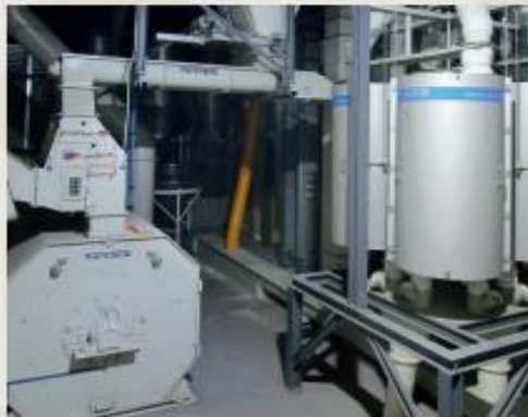
Avenal Racoos Site in Portugal: Preparation of compounds for Petfood. GD 20 Module with Plansifter (Grinding concept V3)
